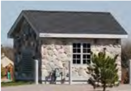
Figure 8. Pumping Station Example Imagery
