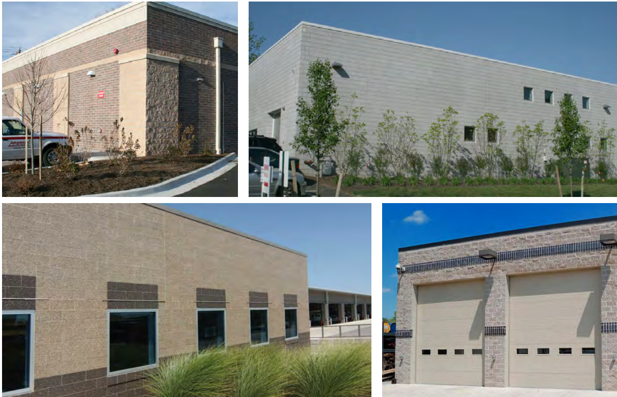
Figure 19. Maintenance and Utility Building Example Imagery
