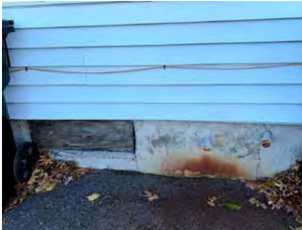
Cracked foundation (left); lack of yard maintenance, car parked on grass, facade wear and tear, and trash in the yard (right).
