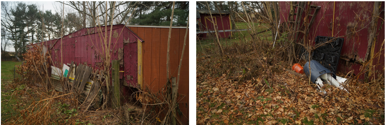
Figure 13. Lot 5: Improperly stored materials
