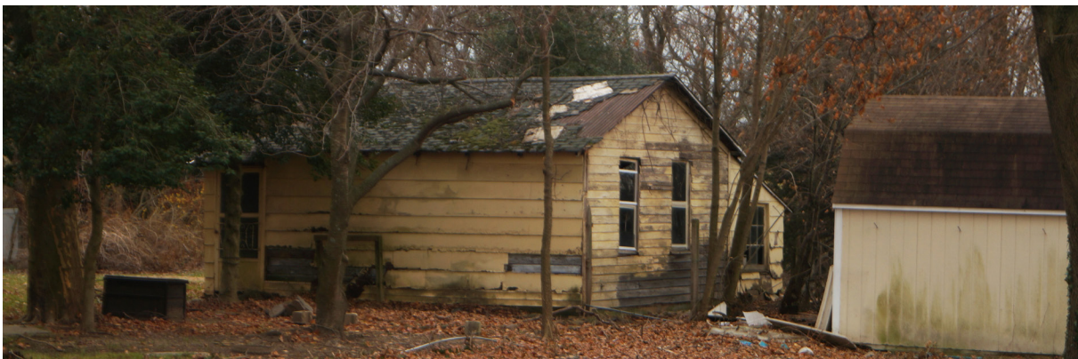
Figure 5. Lot 4.02: Dilapidated Accessory Building
