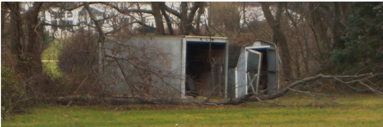
Figure 4. Lot 4.01: Broken Shed and Storage Unit
