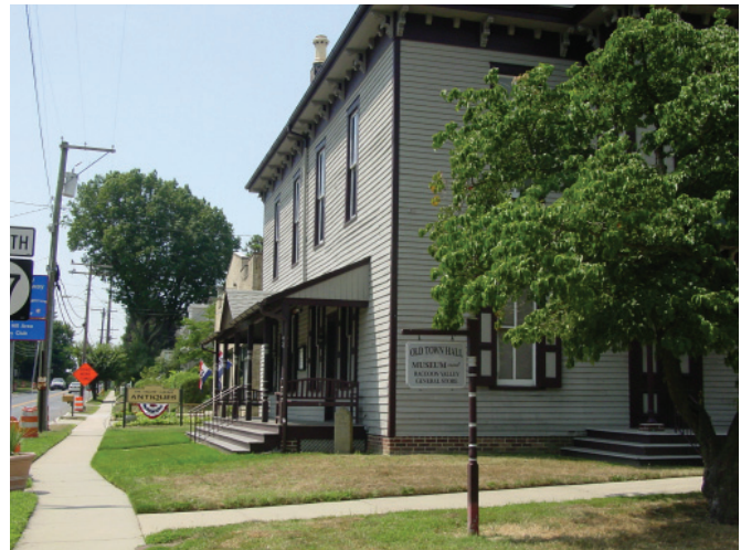
Commercial use along Main Street (top); View south from the intersection of Main and Spicer Streets (bottom)
