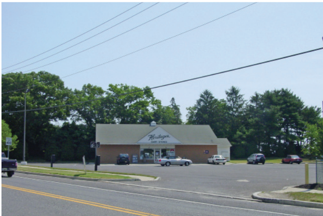
Vacant structure at the intersection of Main Street and Breakneck Road (top); Commercial use located across Breakneck Road from Site 4 (bottom)
