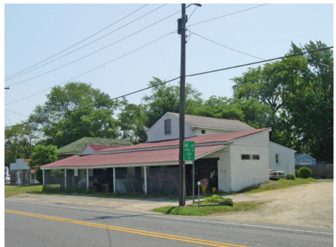
Single-family dwellings along Main Street (top and middle); Accessory storage uses along Main Street (bottom)
